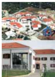
Provider of permanent and temporary accommodation for people with intellectual disabilities Centar za rehabilitaciju "MIR", Kaštel Novi www.centar-mir.hr
